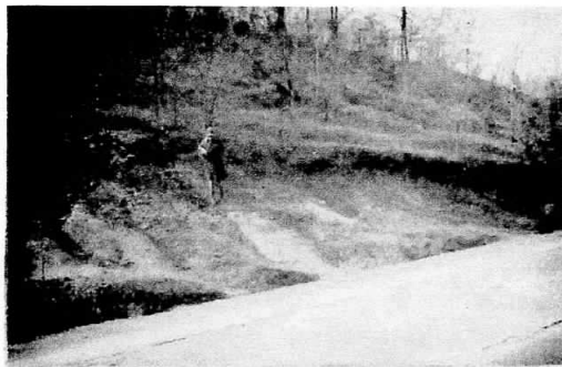
FIG. C SOUTH SIDE, HIGHWAY 36 ROADCUT WEST OF MONTEZUMA, INDIANA
