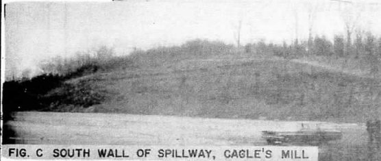
FIG. C SOUTH WALL OF SPILLWAY, CAGLE'S MILL
