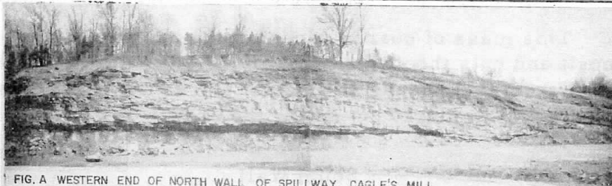
FIG. A WESTERN END OF NORTH WALL OF SPILLWAY, CAGLE'S MILL
